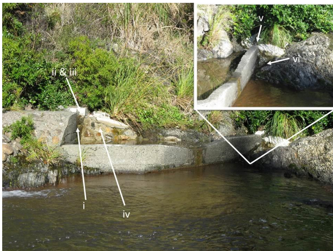
Figure 38. Step-pool fish pass on true left of the Maitai South Branch weir, following remediation work. Numbered arrows indicate remediation undertaken, with numbers referring to the points outlined above. Note: river flow in this image is substantially lower than in Figure 36.
