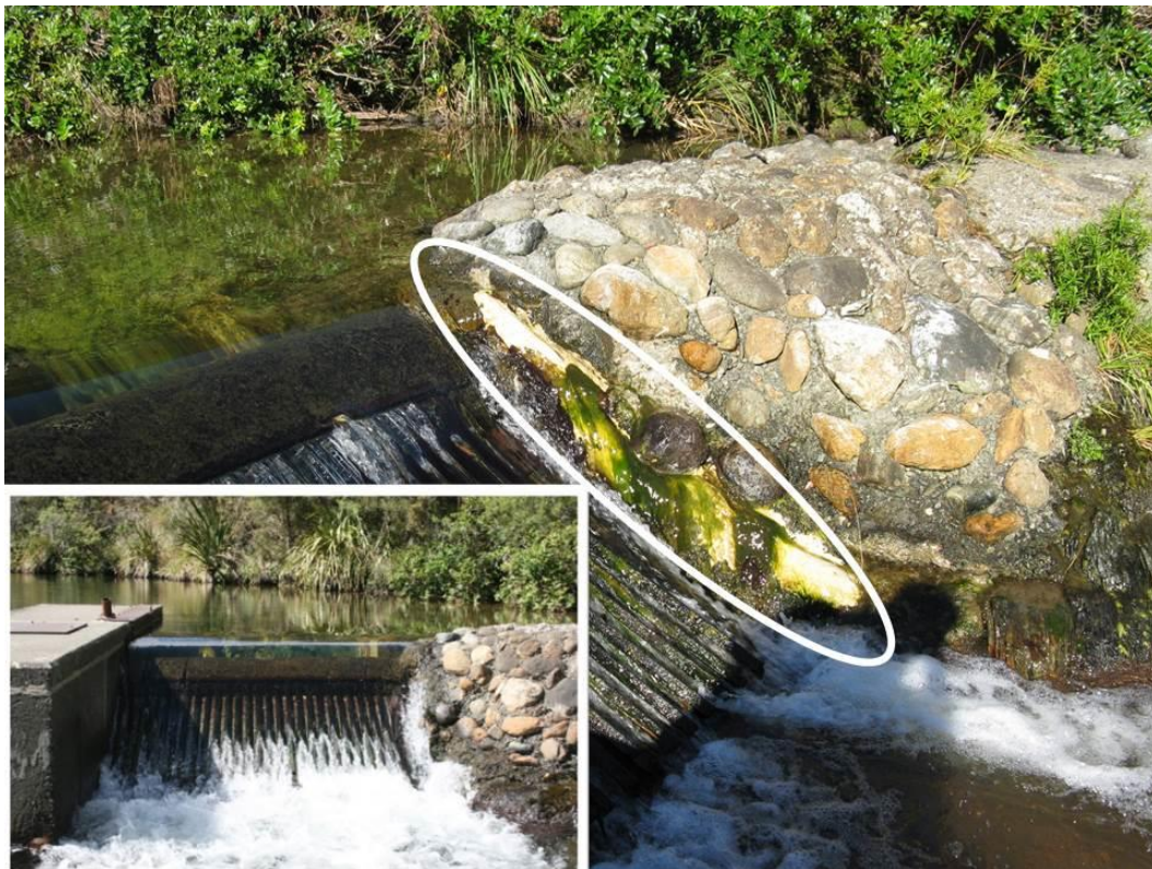
Figure 39. The water intake screen in the Maitai South Branch weir, showing the smooth wetted margin constructed with epoxy cement as part of the remediation works (highlighted within the white oval). Insert shows the screen prior to remediation.
