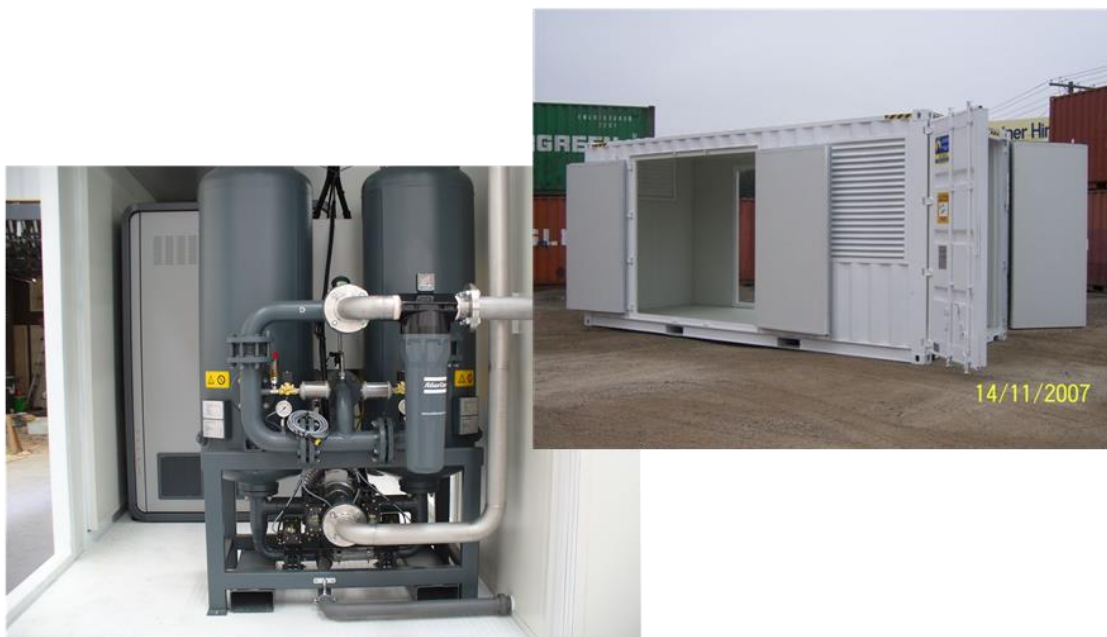
Figure 51. Examples of temporary container buildings used for housing destratification compressor systems.
