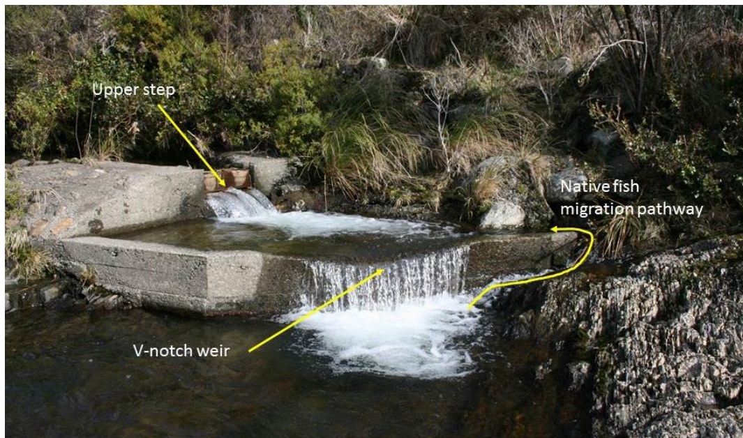
Figure 37. Step-pool fish pass on true left of the Maitai South Branch weir, prior to remediation work.
