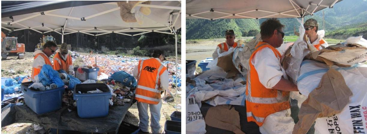
**Figure 3-15: Material being separated into its individual categories**
